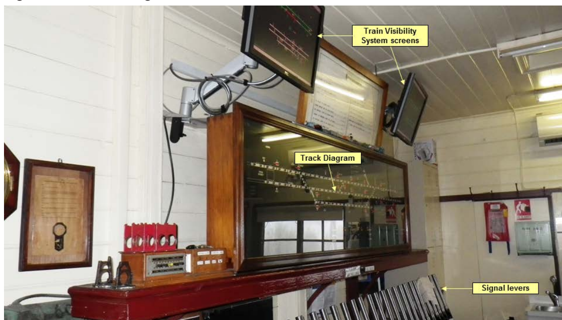
Figure 5: Katoomba signal box
